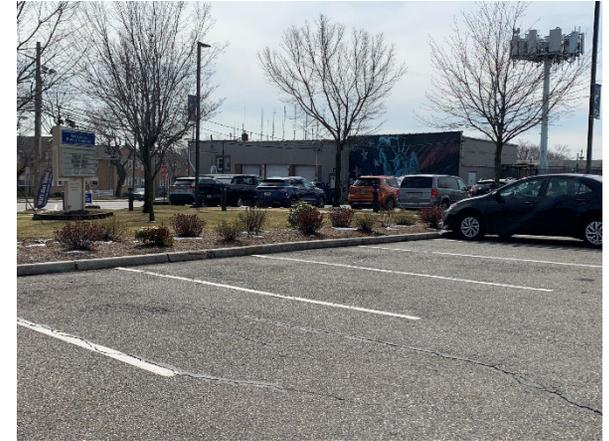
Parking spaces in the parking lot to the south of the building can be converted to porous pavement to capture and infiltrate stormwater runoff from the parking lot. A rain garden can be installed southeast of the parking lot to capture, treat, and infiltrate stormwater runoff from the pavement. Downspout planter boxes can be installed nearby the building entrance to capture the rooftop stormwater runoff.
